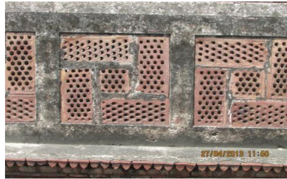
Figure 46: Terracotta Grills at parapet wall of D/747 (Source: Authors)
